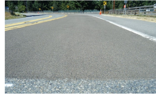
High Friction Surfacing
